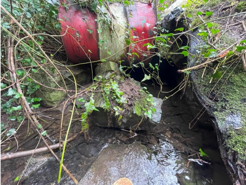
Figure 1.5: Outlet of upstream culvert (Culvert 1) under Baldonnel Road
